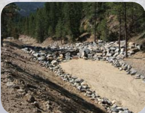
A sediment trap, which reduces metals and sediment flowing from orphan mine sites, is ready for clean out.
