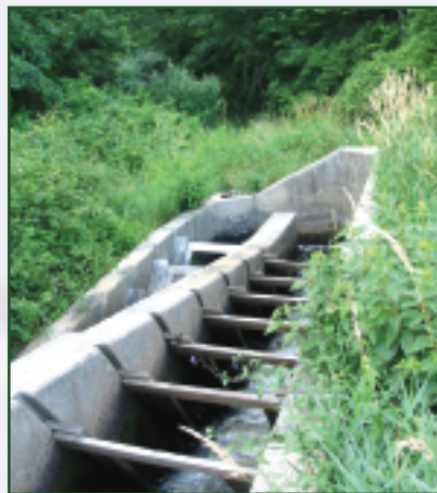
Fish ladder at Bradford Dam will help restore migratory fish runs. (Wood-Pawcatuck Watershed Association)
