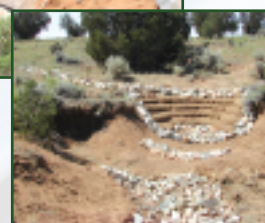
Jute bag structures help stop erosion and the advance of headcuts.
