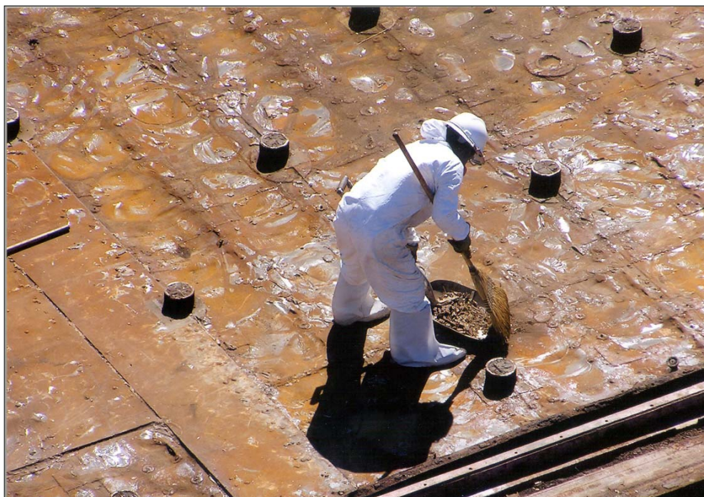
Photo courtesy of Laura S. Johnson Worker sweeping debris during flight deck removal onboard the ex-USS Oriskany.
