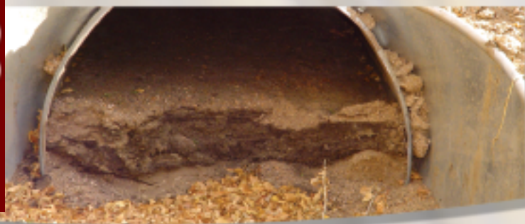
Post-fire erosion nearly fills this culvert with sediment.
