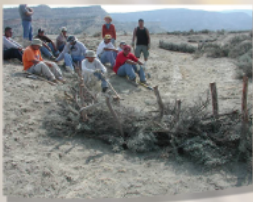
Jemez Pueblo ranchers constructed a series of post and wicker weirs using locally available juniper branches and sagebrush.
