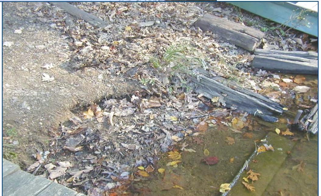
Example of shoreline erosion and dilapidated bulkheading
