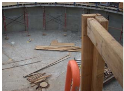
Water treatment facility expansion in Buckeye, Arizona. (EPA OIG photo)
