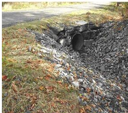
King Hill Road—After
