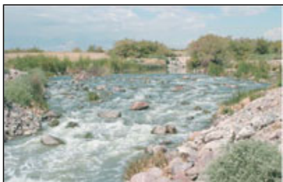
Weirs are low dams designed to reduce streambed erosion by flattening the slope of the channel and slowing flows. Many weirs are constructed of confined rock riprap, providing a somewhat natural look (left). Other structures are built with concrete, resulting in a more engineered look (right). Weirs, wetland restoration, and invasive vegetation removal helped reduce total suspended solids (TSS) concentrations in lower Las Vegas Wash and led to its removal from the Nevada 303(d) list in 2004.
