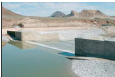
Weirs are low dams designed to reduce streambed erosion by flattening the slope of the channel and slowing flows. Many weirs are constructed of confined rock riprap, providing a somewhat natural look (left). Other structures are built with concrete, resulting in a more engineered look (right). Weirs, wetland restoration, and invasive vegetation removal helped reduce total suspended solids (TSS) concentrations in lower Las Vegas Wash and led to its removal from the Nevada 303(d) list in 2004.
