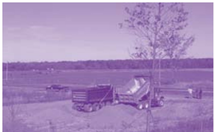
Dump truck with deposits of crushed concrete ready for use.
