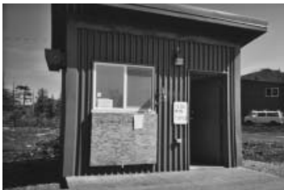
Entrance to the Klawock Transfer Station.
