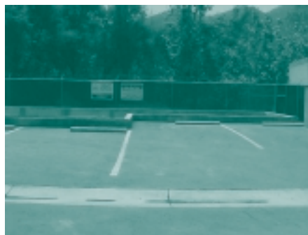
Front view of the waste unloading area at the Tule River transfer station.
