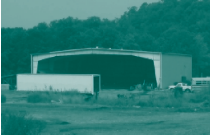
The Eastern Band of Cherokee Indians' enclosed transfer station building.
