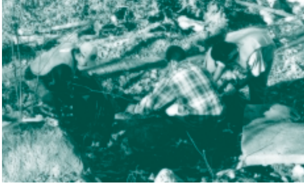
Contractors clean up an illegal dump site on White Earth Reservation.
