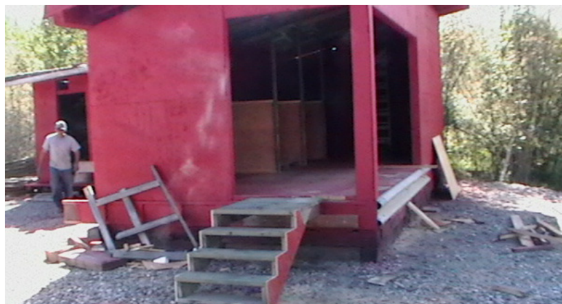
Construction of the Nenana Recycling Center.
