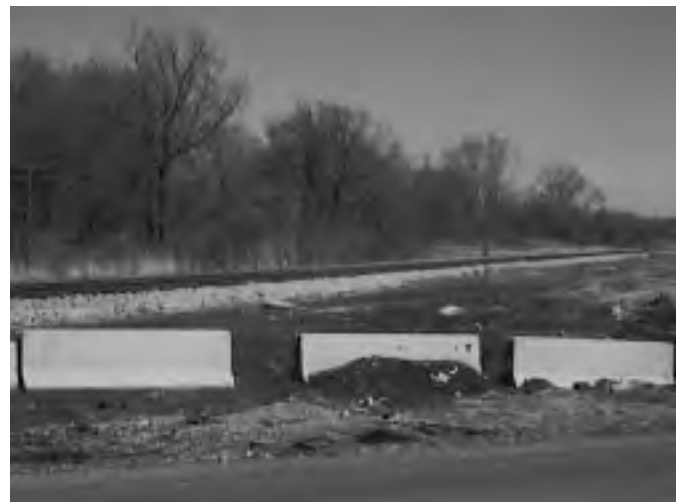
Concrete barriers preventing access along railroad right-of-way
