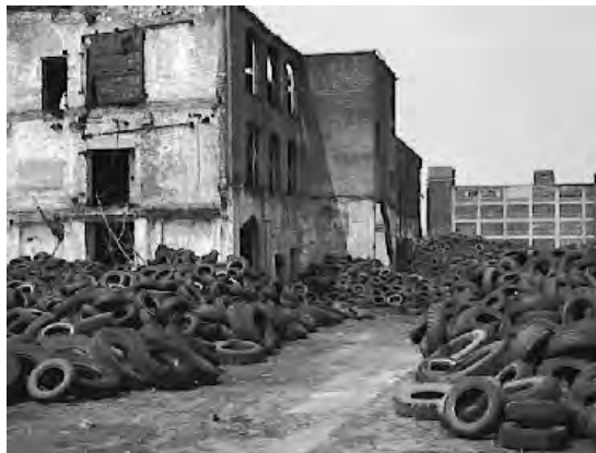
Illegally dumped tires in and around an abandoned warehouse
