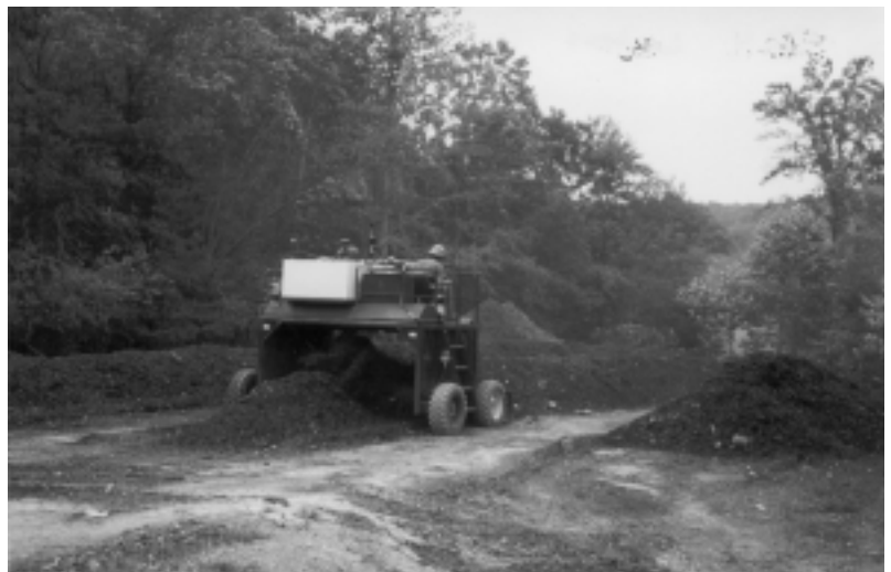
Eastern Band of Cherokee Indians' composting operations. Top: windrow turner aerates the piles to increase decomposition. Bottom: watering the piles helps maintain the proper moisture levels.
