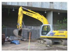
Field observers should watch that the area is roped off during the time the crew is crushing empty containers and that containers are empty.
