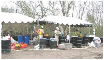
protective clothing worn by all pad workers, this area requires respirators and splash aprons. In addition, workers should attempt to bulk and secure all material received at this pad prior to leaving for the night.
