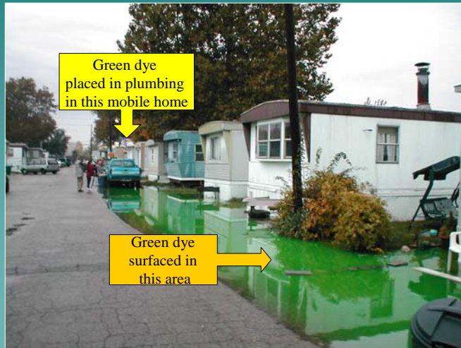
Illicit Discharge Elimination Program, Macomb County, MI.
