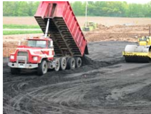
Figure 2. Compacting fill material at the project site.
