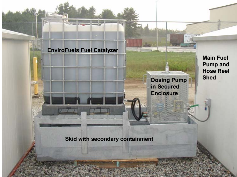
Figure 1-2. EnviroFuels Tote, Dosing Pump, and Skid
