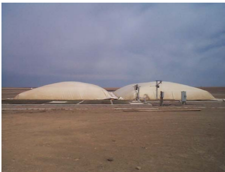
Figure 1-3. Colorado Pork Anaerobic Digester
