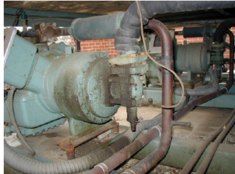
2 compressors operating in series (refrigerant charge of 70 and 69 lbs R-22)
