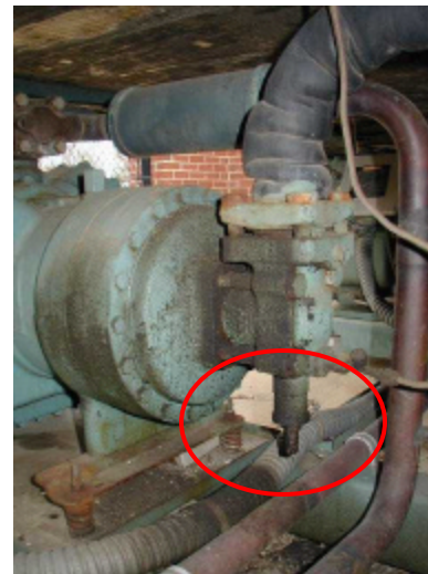
2 compressors operating in series (refrigerant charge of 70 and 69 lbs R-22)
