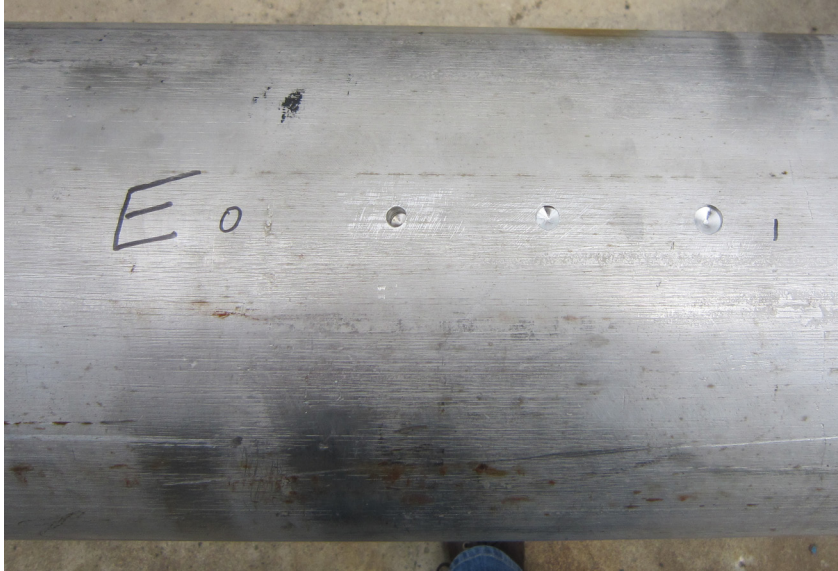
Figure 6-4. Uninsulated Pipe Sample 2 simulated defects.
