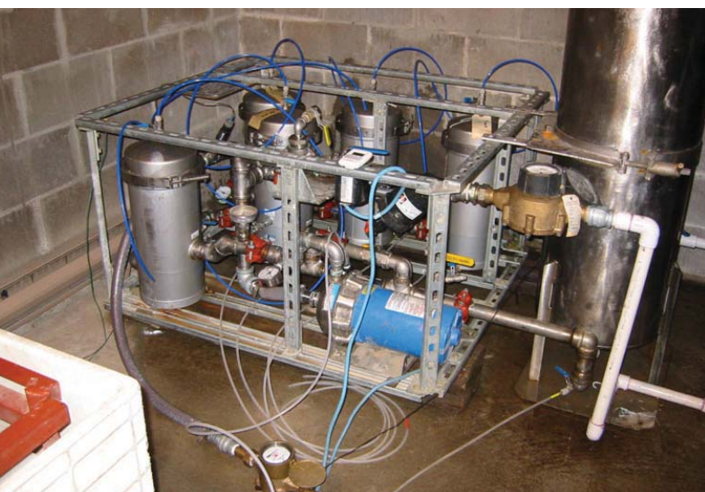
Two of the ETV-verified arsenic drinking water treatment technologies
