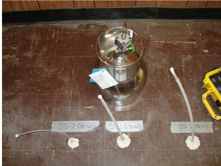
Figure 9. Installed SS Sampling Points (Photo courtesy Dr. Thomas McHugh, GSI.)
