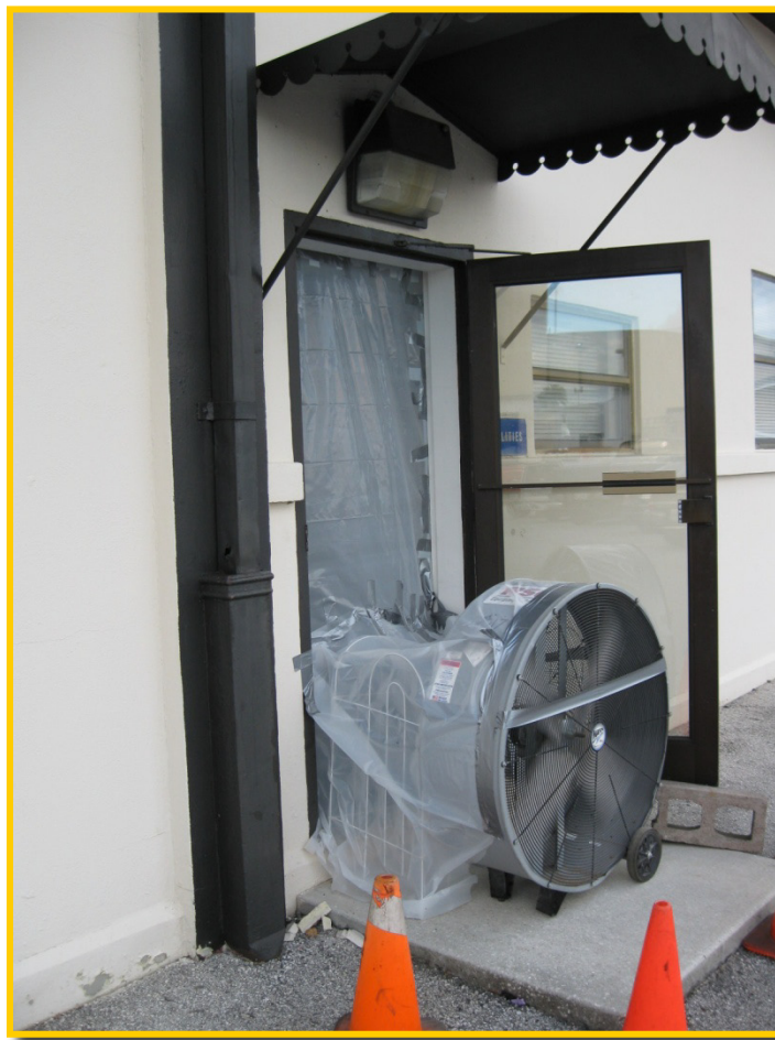
Figure 3. Fan Installed in Building Doorway to Manipulate Building Pressure (Photo courtesy Dr. Thomas McHugh, GSI.)
