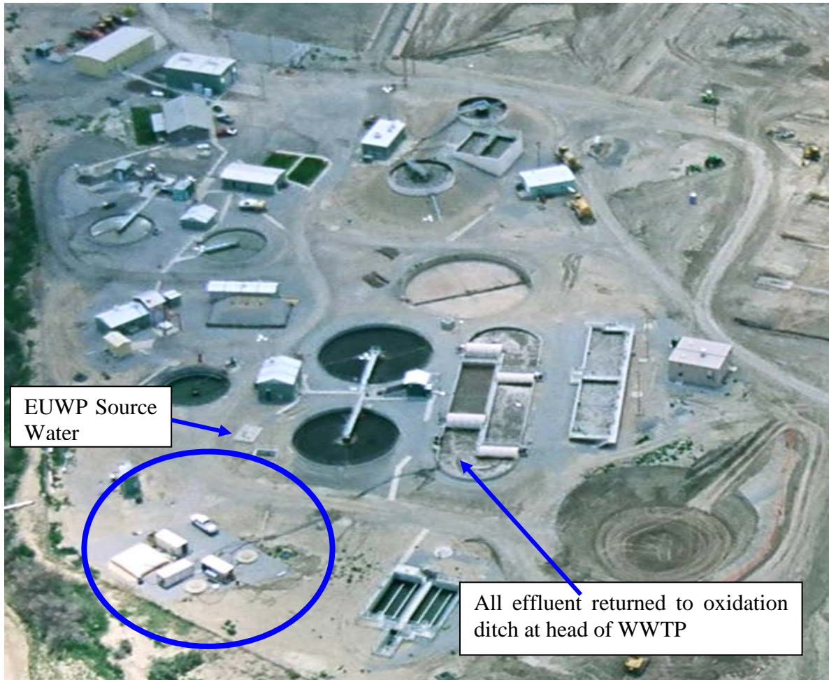
Figure 1-2. Gallup Wastewater Treatment Plant with EUWP indicated by the circle.
