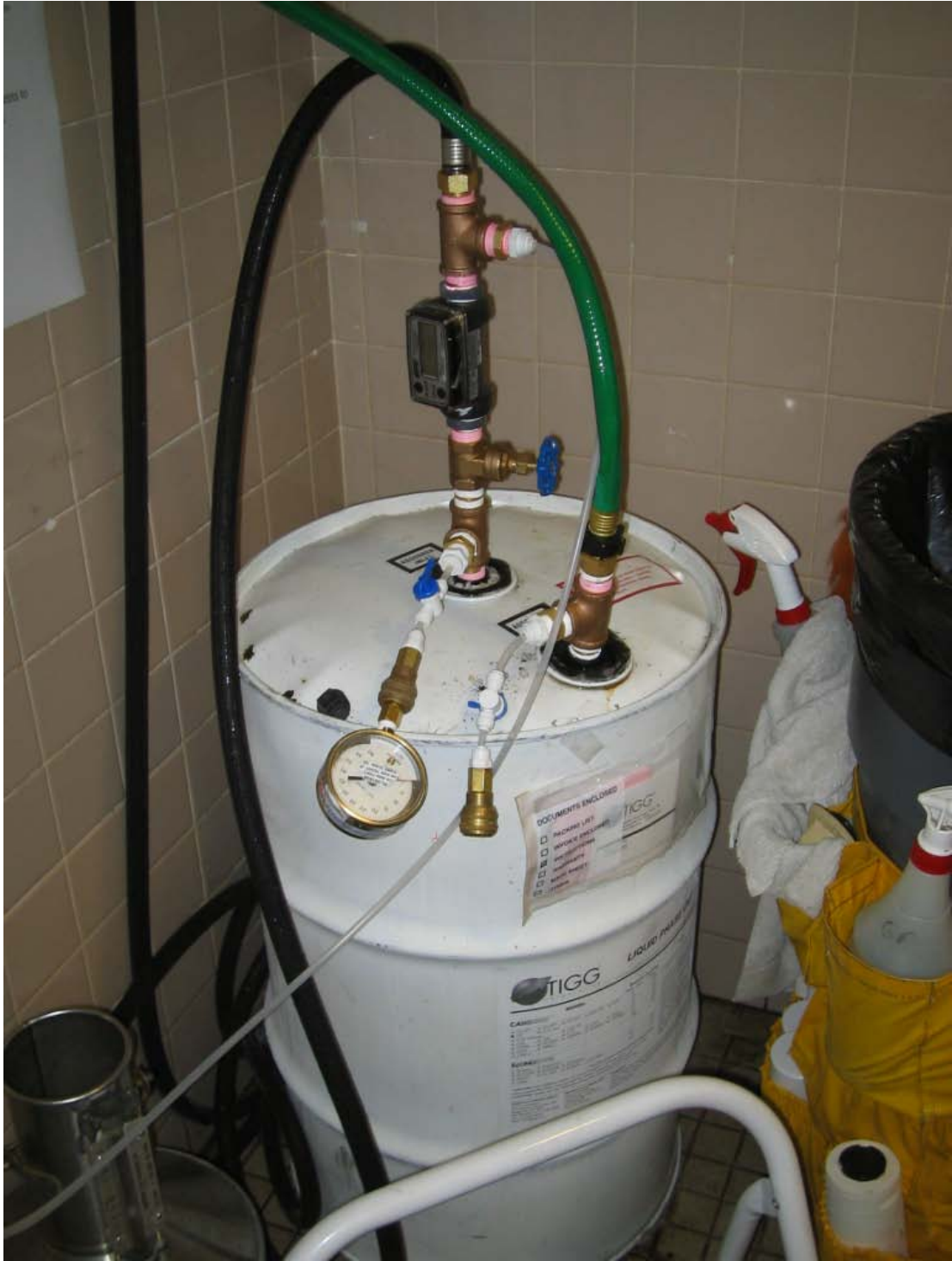
Figure 2-1. Photo #1 of the Brimac pilot unit.
