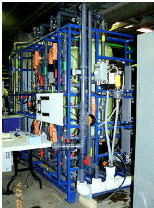
Photo 2. Side view of the Kinetico SW224 Filter System at the University of Minnesota.
