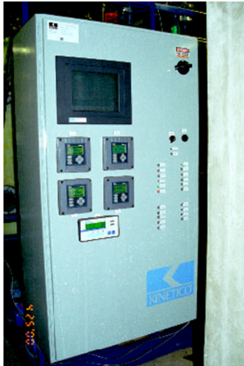
Photo 1. Front view of the was Kinetico SW224 Filter System at the University of Minnesota
