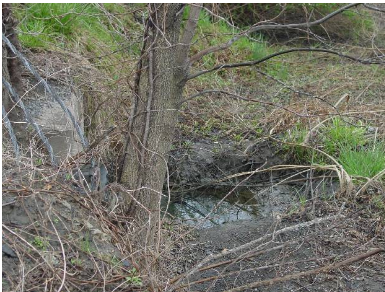
Figure 3-5. Outlet sampling location for 15-inch reinforced concrete storm drain pipe.
