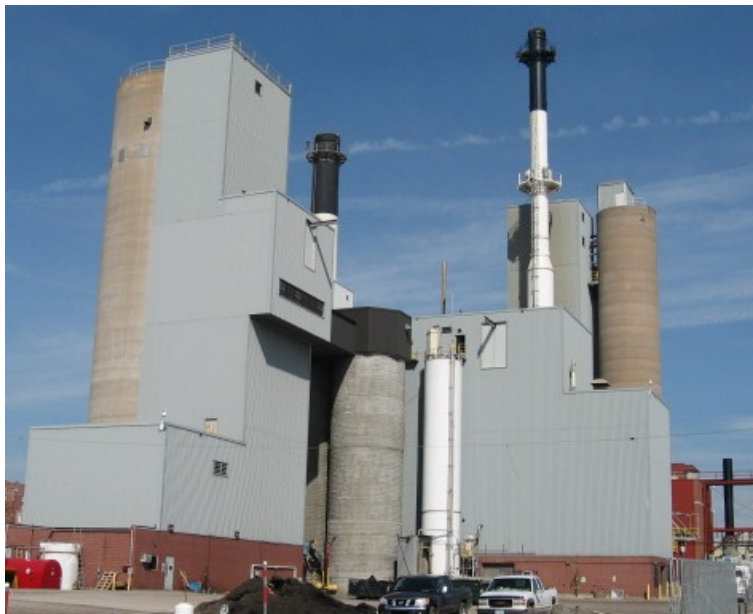
Figure 2-1. The University of Iowa Main Power Plant
