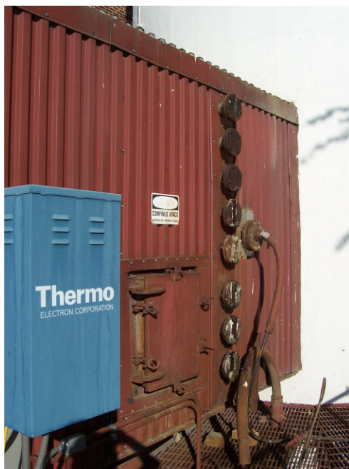
Figure 2-2. Test Port Locations for Boiler 10
