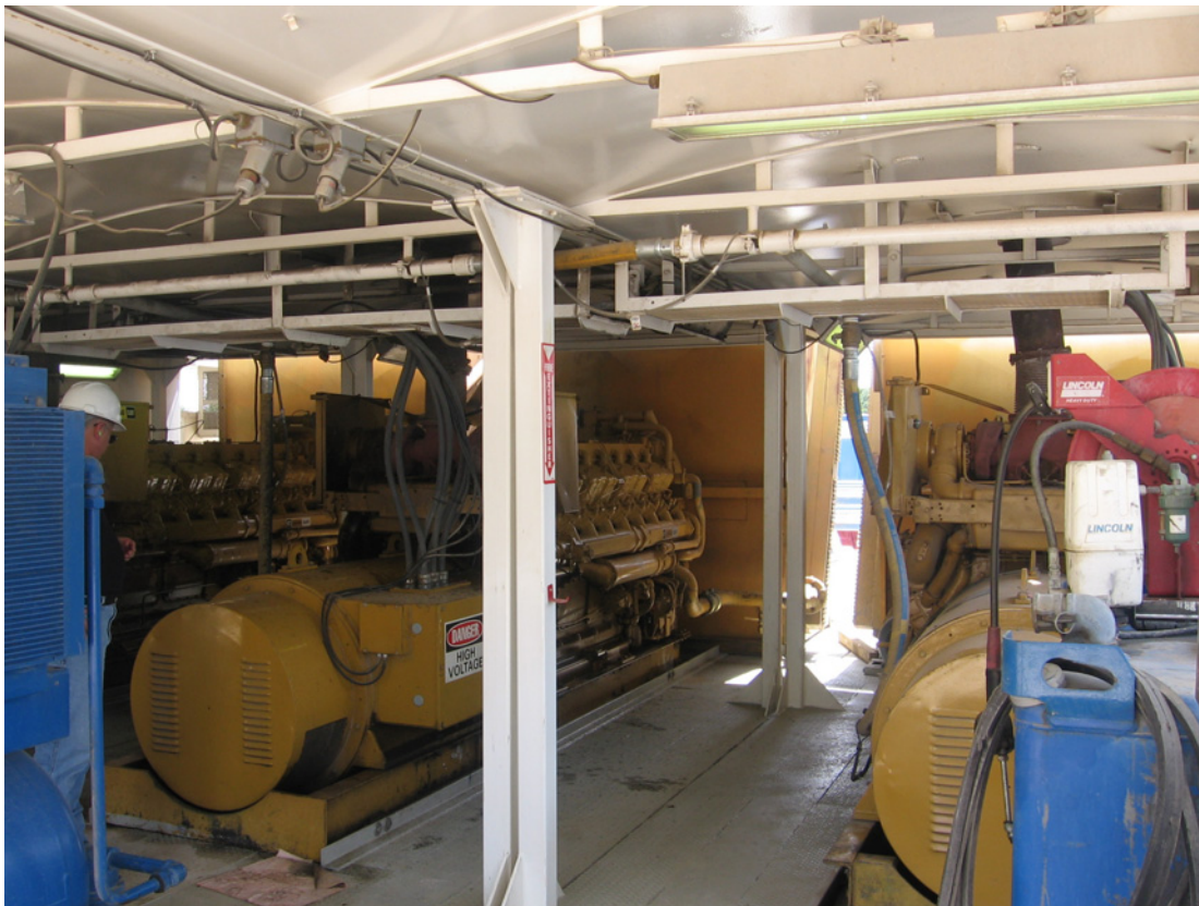
Figure 1-2. Cat 399s on Nabors 313 Rig
