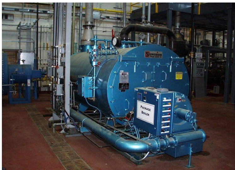
Figure 3-1. Wetback Scotch Marine Package Boiler
