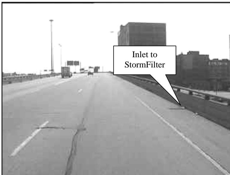
Figure 3-3. StormFilter drainage area condition.
