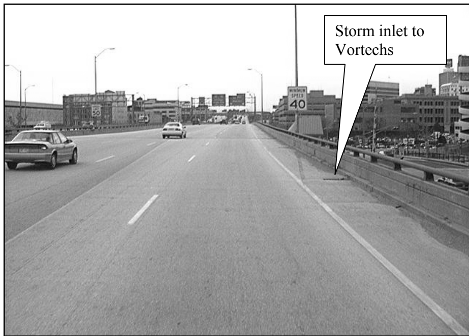
Figure 3-3. Vortechs drainage area condition.
