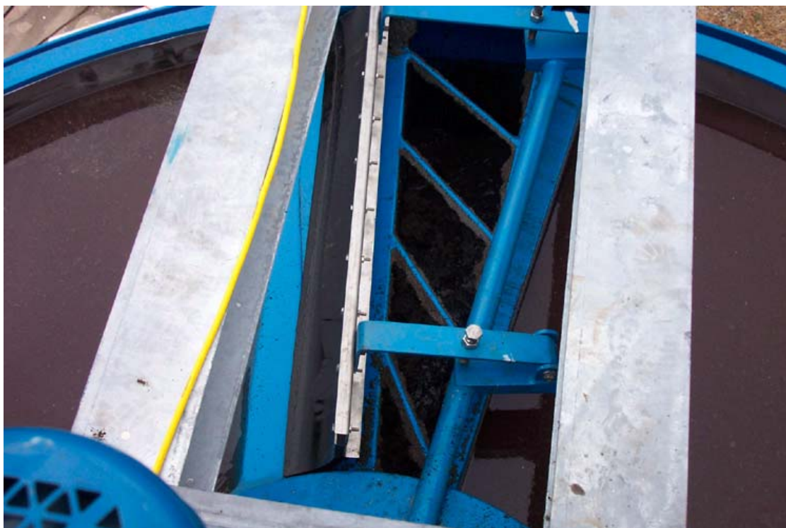
Figure 2-3. Floating solids skimmer box.
