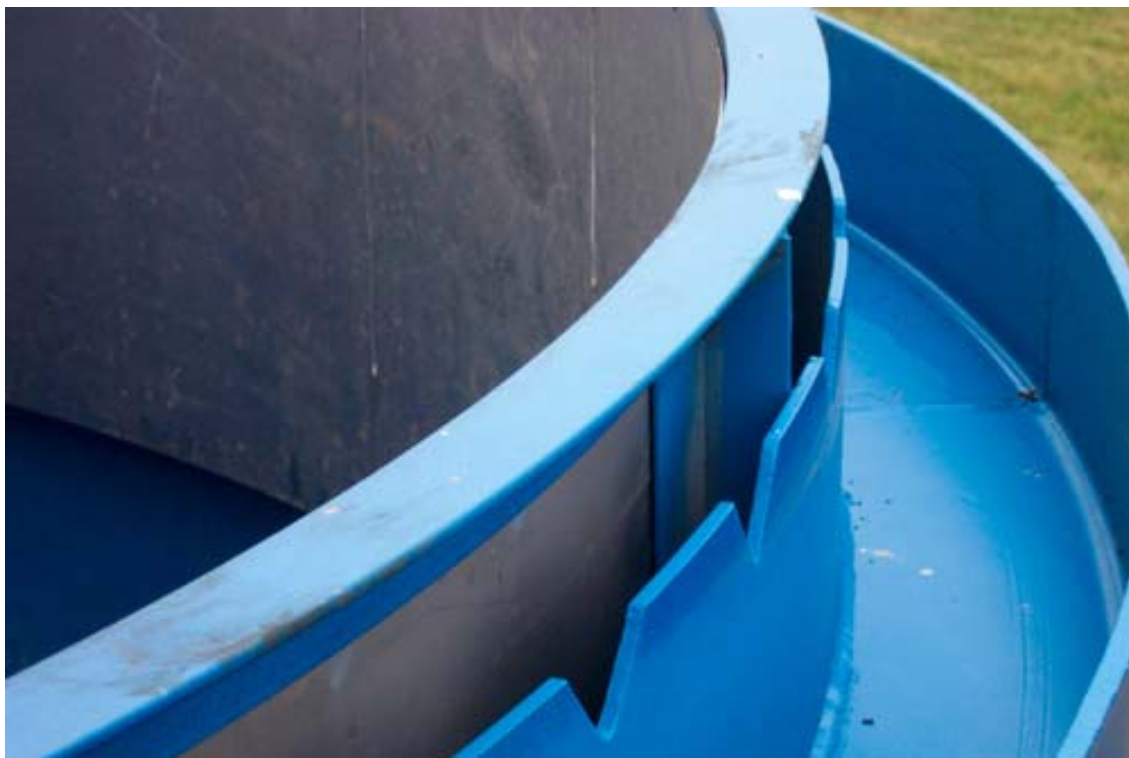
Figure 2-5. Effluent weir and baffle.
