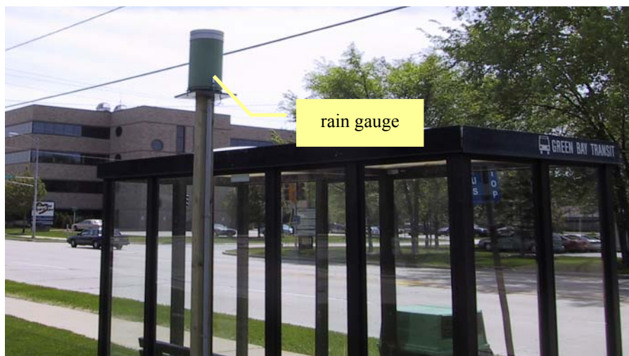
Figure 4-5. View of site rain gauge.
