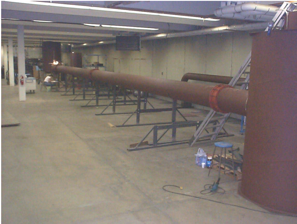
Figure 3-6. The 20-inch simulated sewer (riser-pipe-manhole, right to left).
