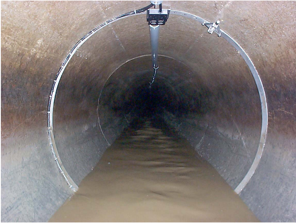
Figure 4-10. ADS 4000 flow meter components.
