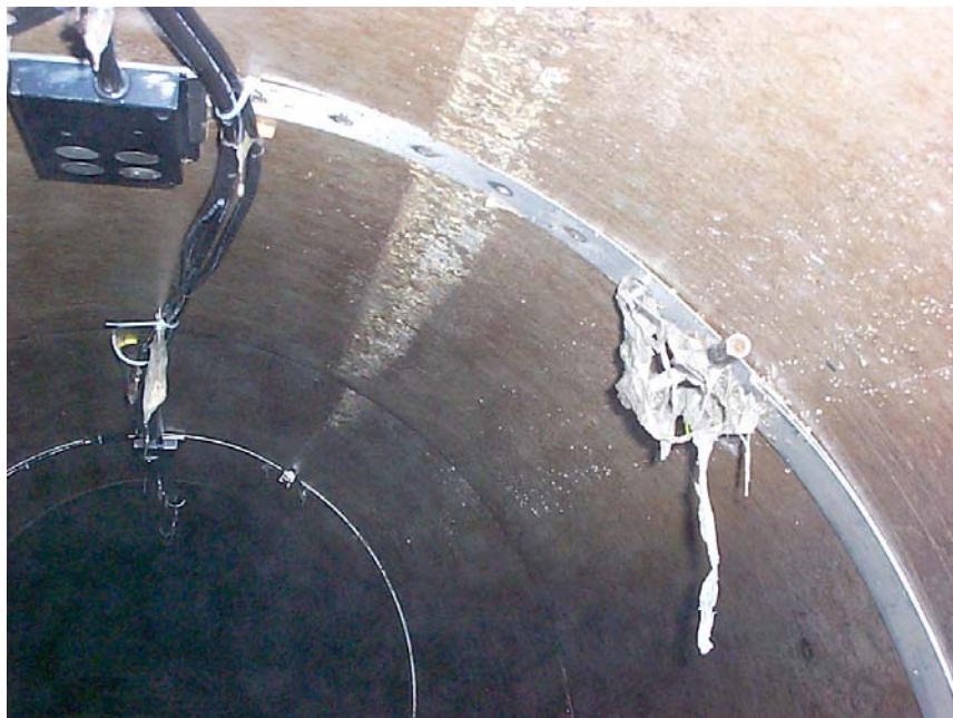
Figure 4-26. Debris accumulation on ADS 4000's bender.
