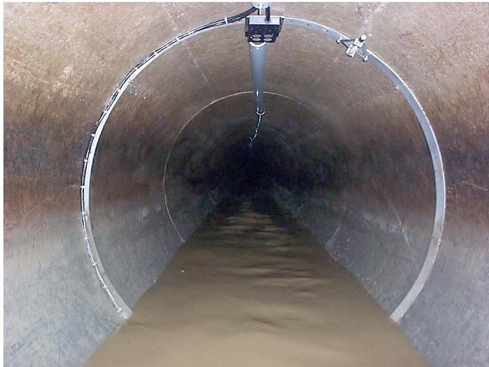
Figure 4-11. ADS 3600 flow meter installed in pipe.
