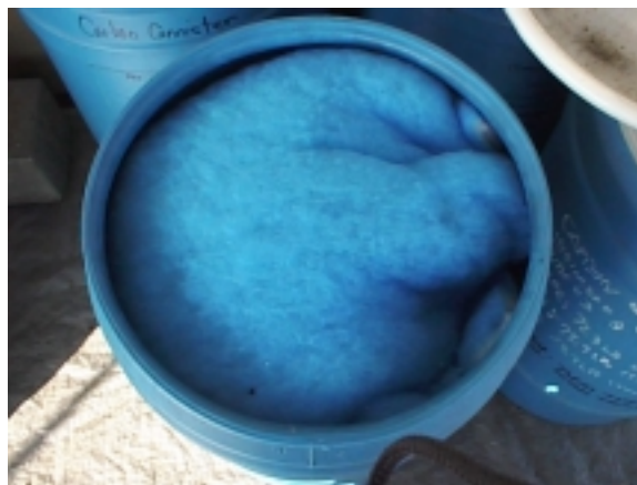
Figure 8 Carbon Filter with Top Removed
