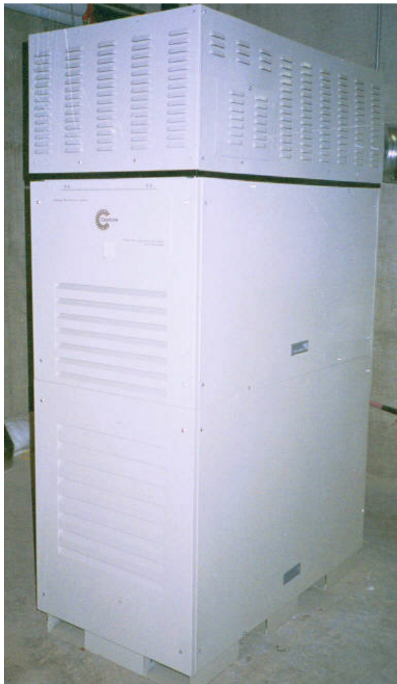
Figure 1-1. The Mariah Combined Heat and Power System
