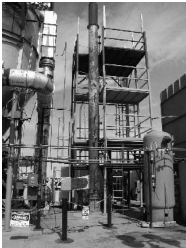
Figure 3-2. TEAD Incinerator Stack
