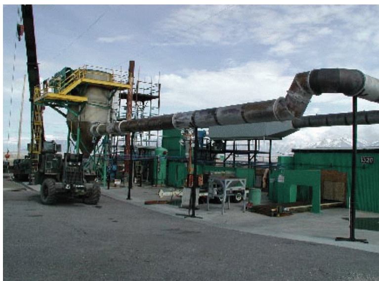
Figure 3-1. Deactivation Incinerator at TEAD
