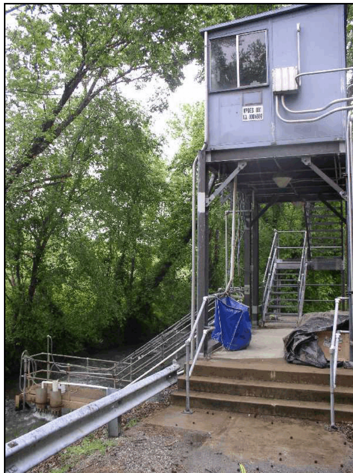
Figure 3-3. Test Site Showing Analyzer Shelter
