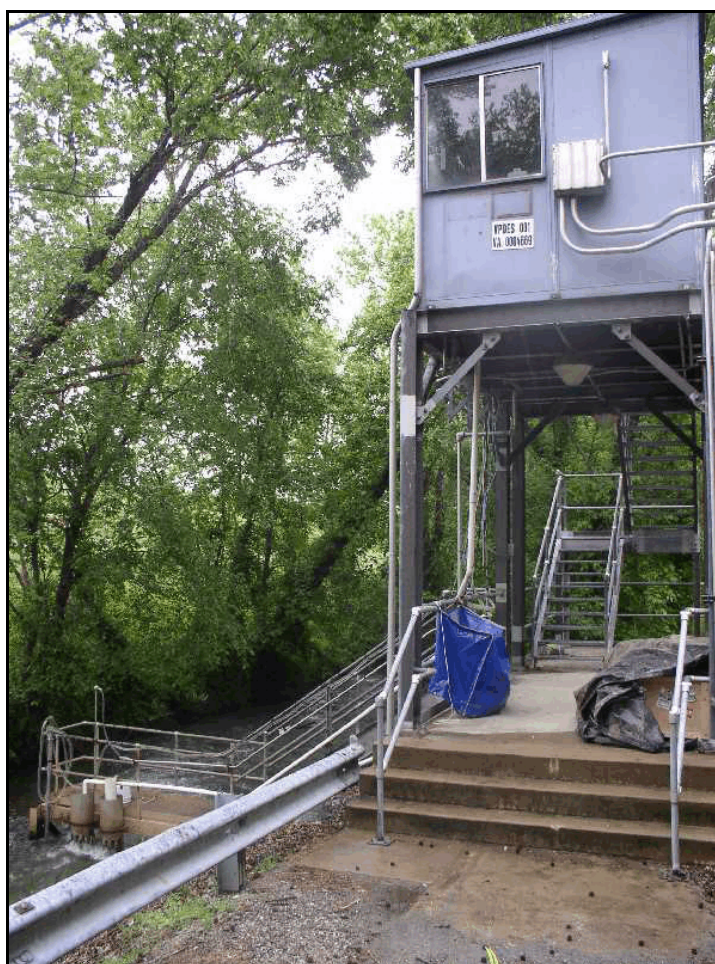
Figure 3-3. Test Site Showing Analyzer Shelter
