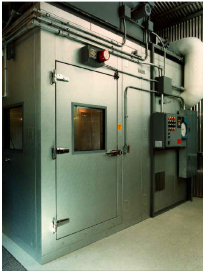
FIGURE 4: Controlled Environmental Atmosphere ("chamber") facility at Building 5507.
