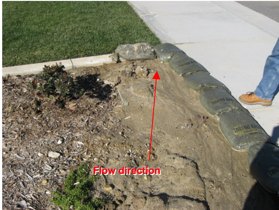
Photograph 9: Sediment accumulated in the down-gradient landscaping
