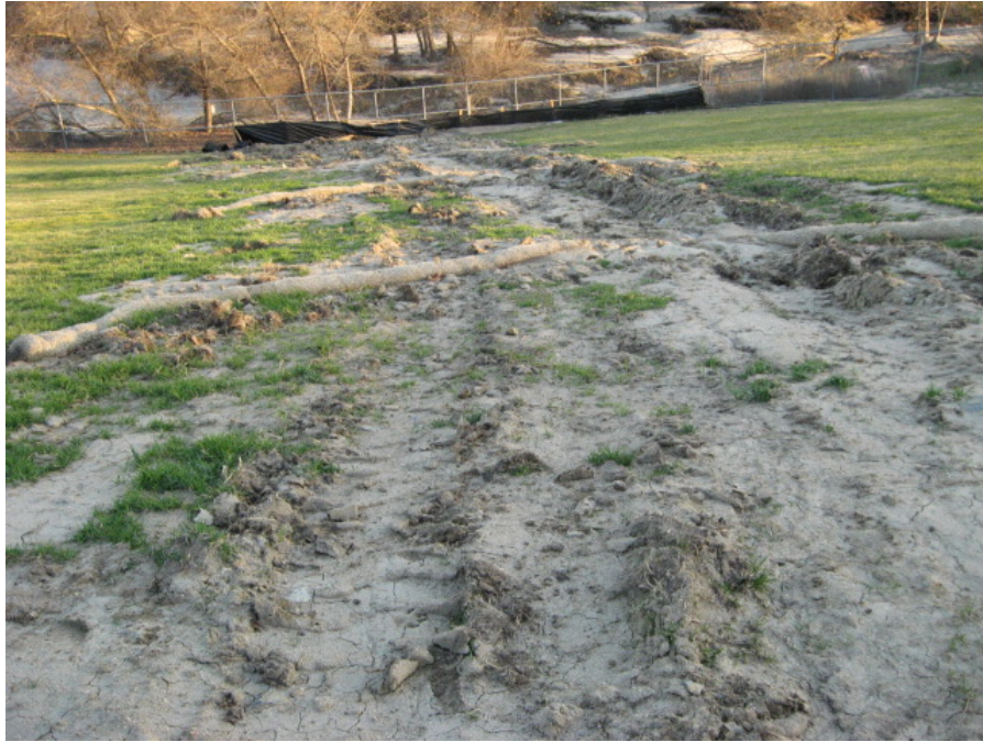
Photograph 1: View of the disturbed slope area at the northern perimeter of the YMCA site
