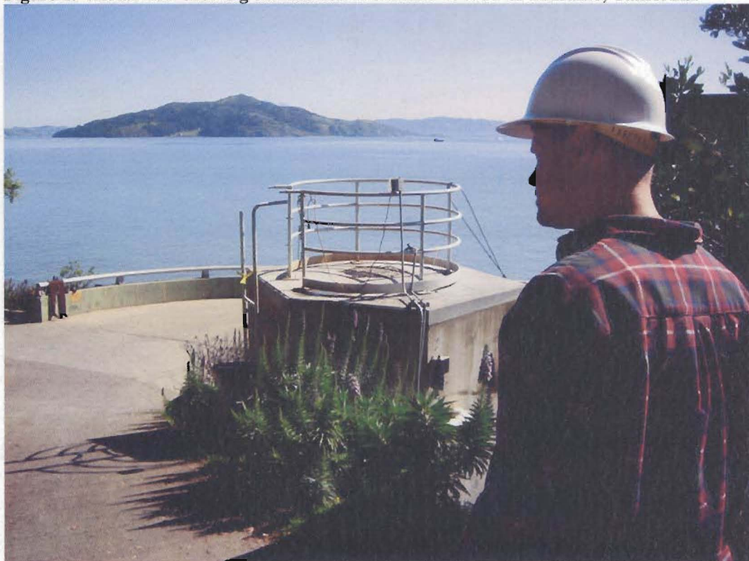
Figure 2: Energy dissipation box
