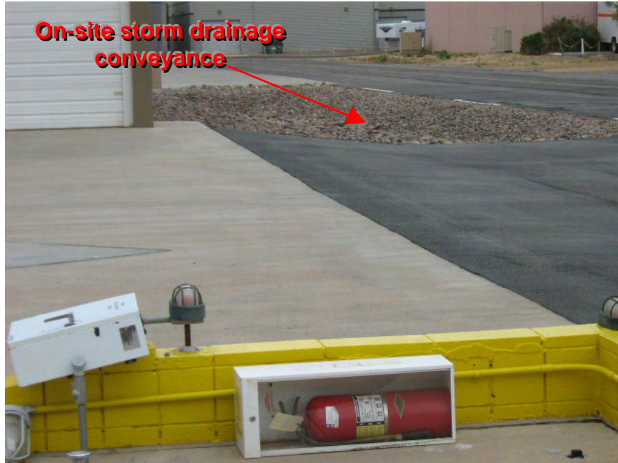
Photograph 5. Scottsdale Airpark – View of Aircraft fueling system located northeast of 7916 East Beck Lane; potential for spills and subsequent conveyance to storm drain system.
