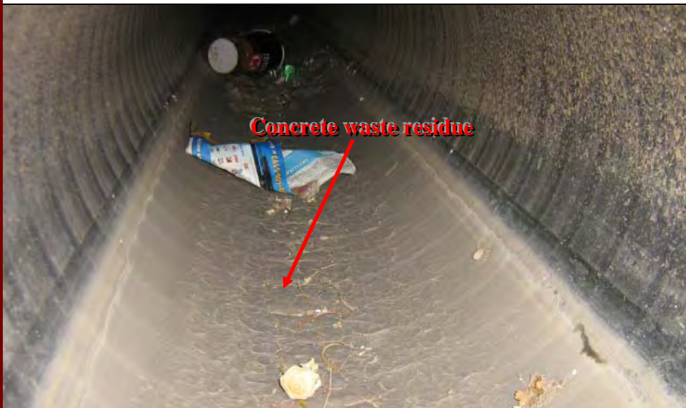
Photograph 3 – View inside outlet pipe shown in previous photographs
