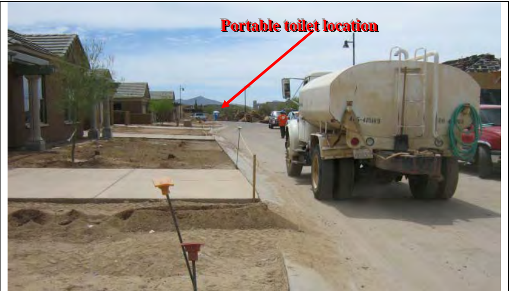
Photograph 10 – View from construction site entrance to the west
