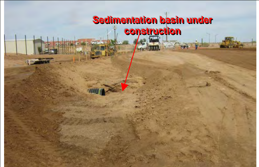
Photograph 2 - Sedimentation basin construction located in the southwest portion of site
