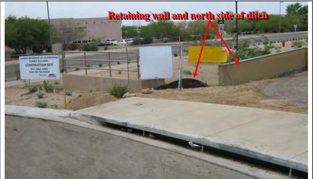
Photograph 6 – View of construction site exit along Williams Drive
