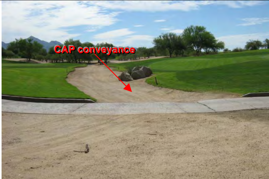
Photograph 1 - Central Arizona Project (CAP) conveyance
