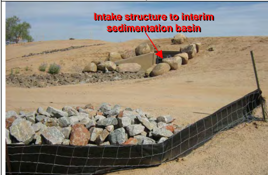
Photograph 7 – Intake structure located in the southeast portion of the site
