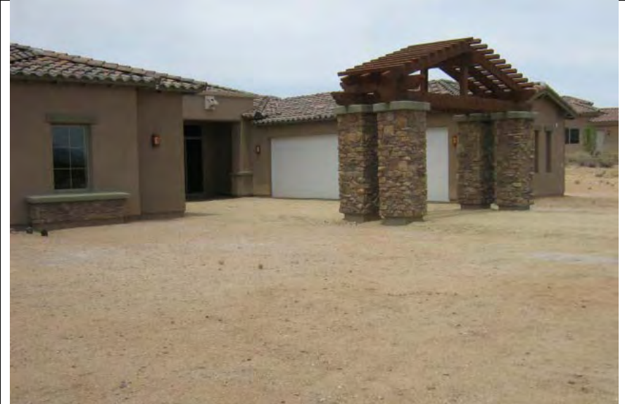
Photograph 2—Constructed home at the center of Lot 64
