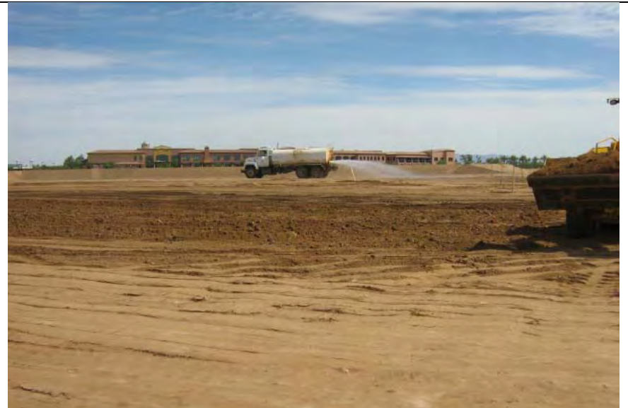
Photograph 6 – Large exposed area in the southeast portion of the site
