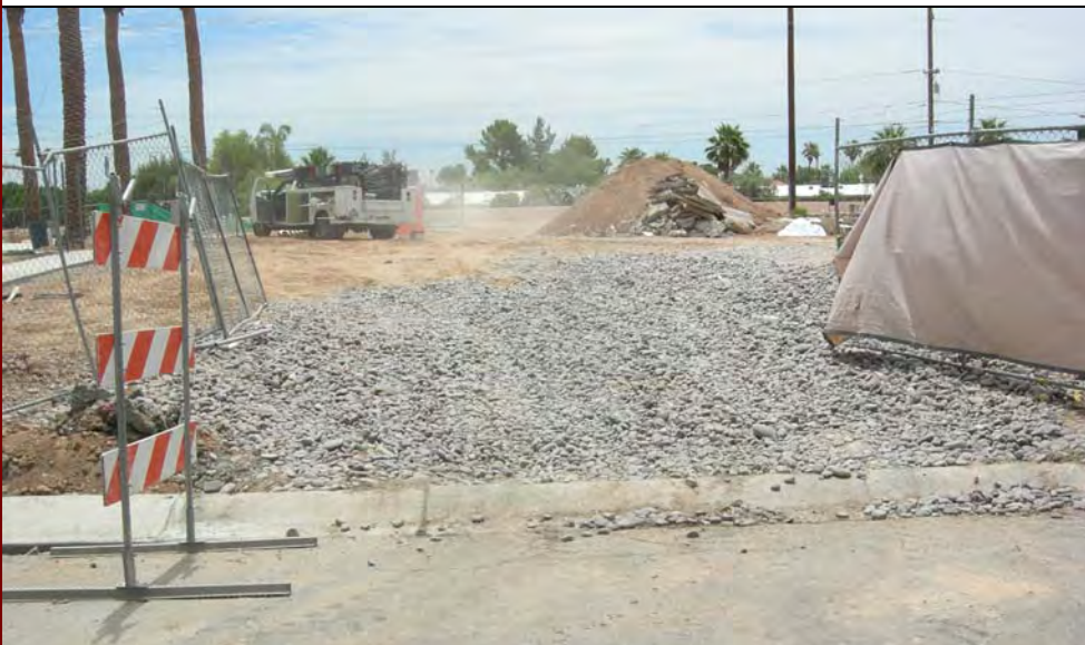
Photograph 3 – View of Phase II construction entrance, facing east.
