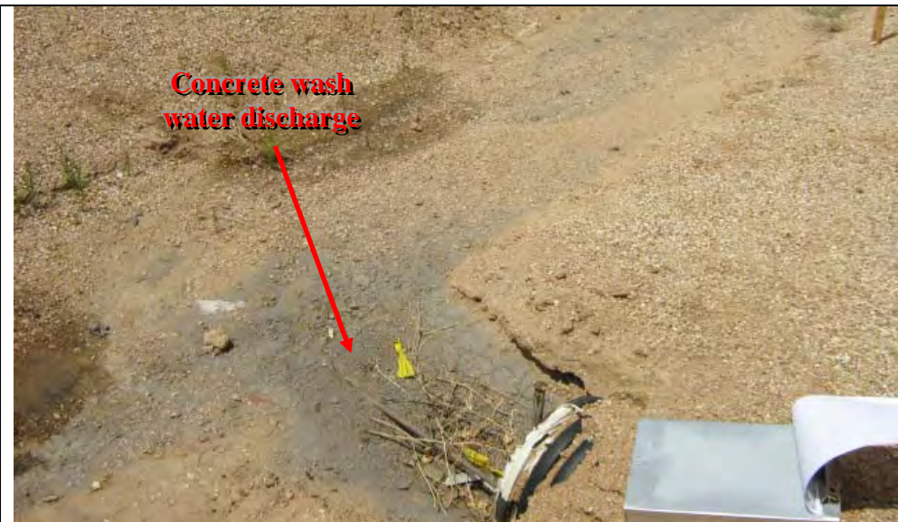
Photograph 2 – Close-up view of outlet shown in Photograph 1
