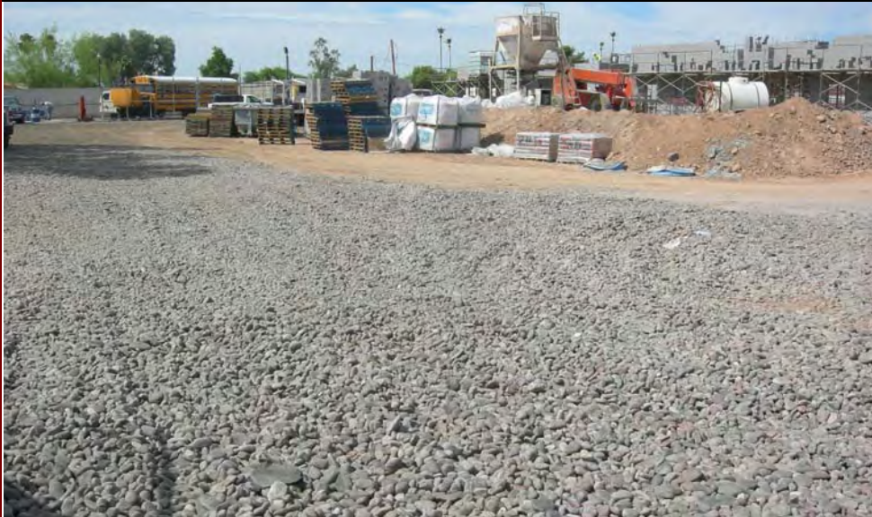
Photograph 1 – View of construction entrance facing south.
