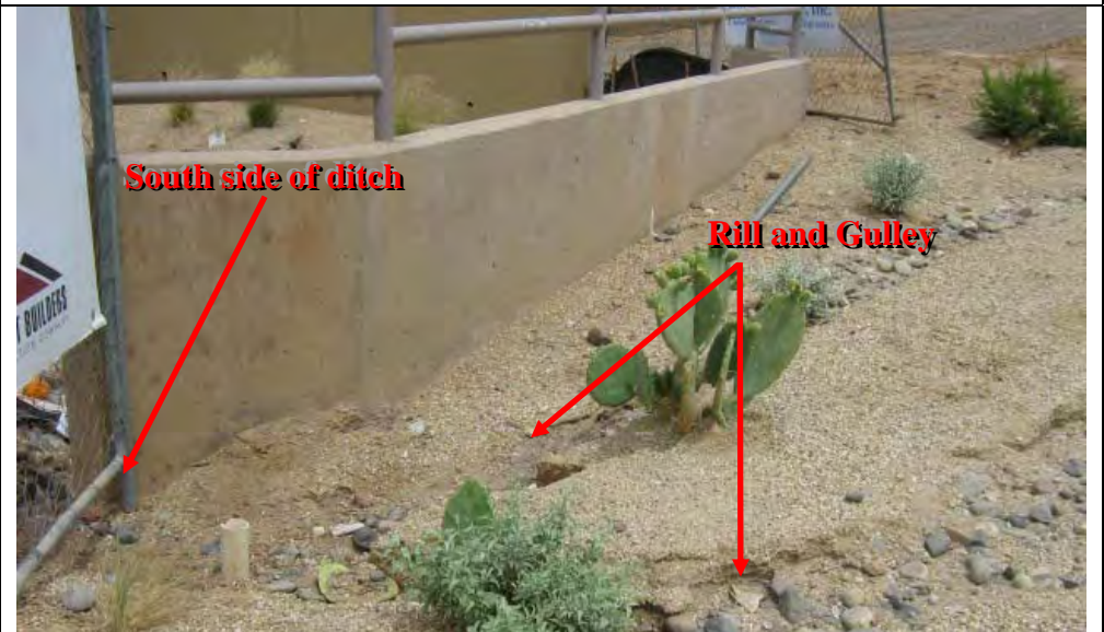
Photograph 8 – Rill and gully pathways on the south side of the drainage ditch
