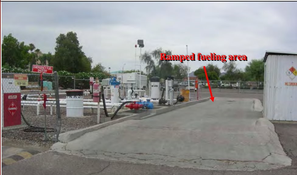
Photograph 3—Landmark Aviation fuel tank area
