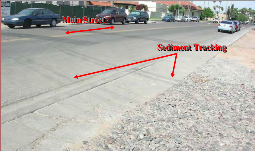
Photograph 3 – View of vehicle tracking onto Main Street, facing northeast.
