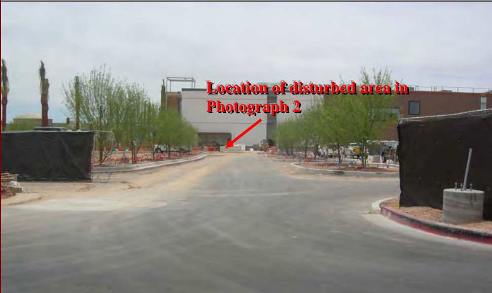
Photograph 3 - View of sediment tracking from the construction entrance at the northeast corner of the site, facing south.
