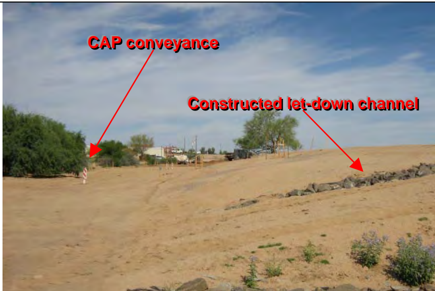
Photograph 3 - Exposed areas up-gradient and down-gradient of the sedimentation basin, adjacent to the CAP
