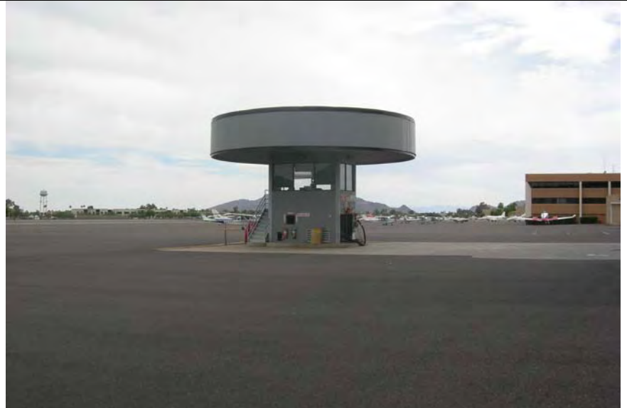
Photograph 2— View of airplane fueling station in front of the airplane hangar from Photograph 1
